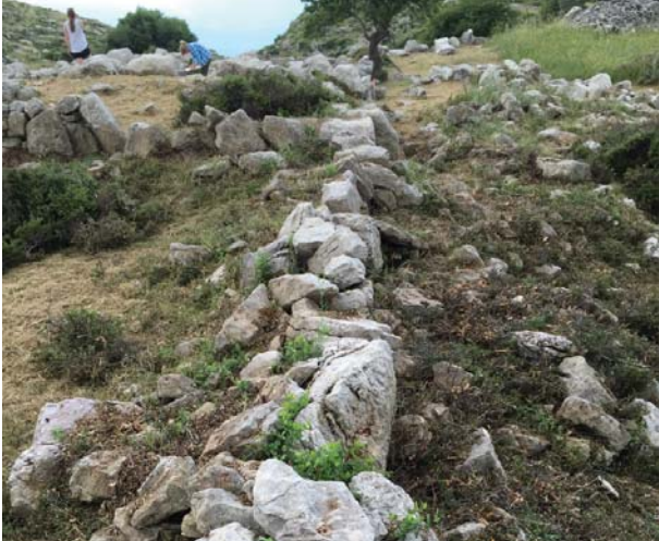
The Bath House area was cleaned and potential new walls of the structure were revealed.
