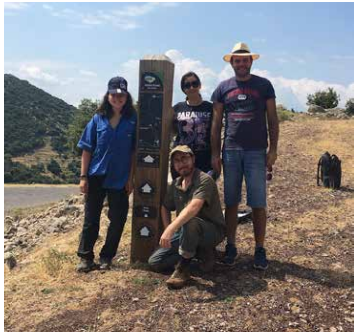
Catherine Skinner, Bucky Stanton, Fani Kazantzi, Vasilis Barkoulas installing trail signs on the Trail of Pan
