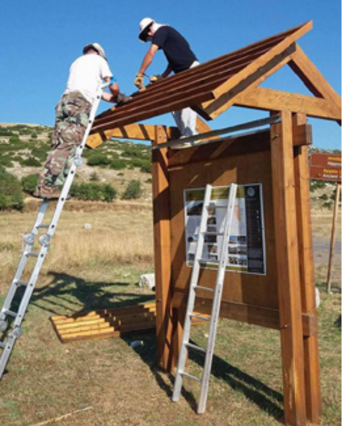
John Keck and Alex Weber install the kiosk roof.
